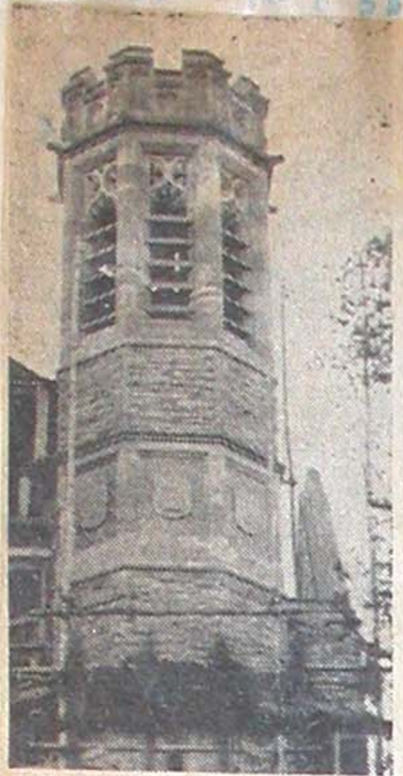
HOW ONE OF THE towers on Bonython Hall looks since the scaffolding has been removed. A photograph taken today.
