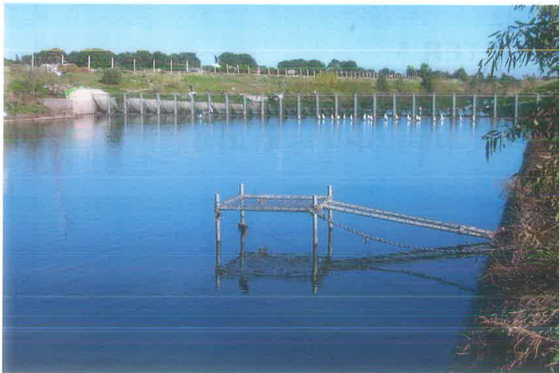
Figure 5-1: The platform in the Morphett Road Sedimentation Pond
