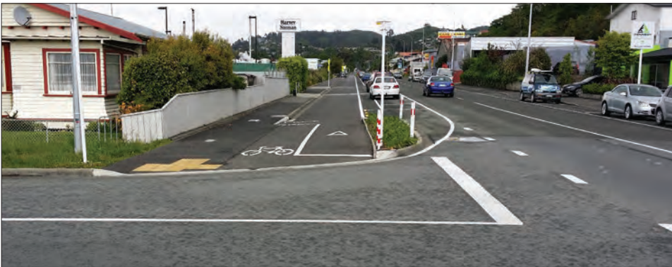
Figure 12.8: A separated cycleway with some ambiguity over side-road priority, in Nelson, New Zealand. (Source: Author.)
