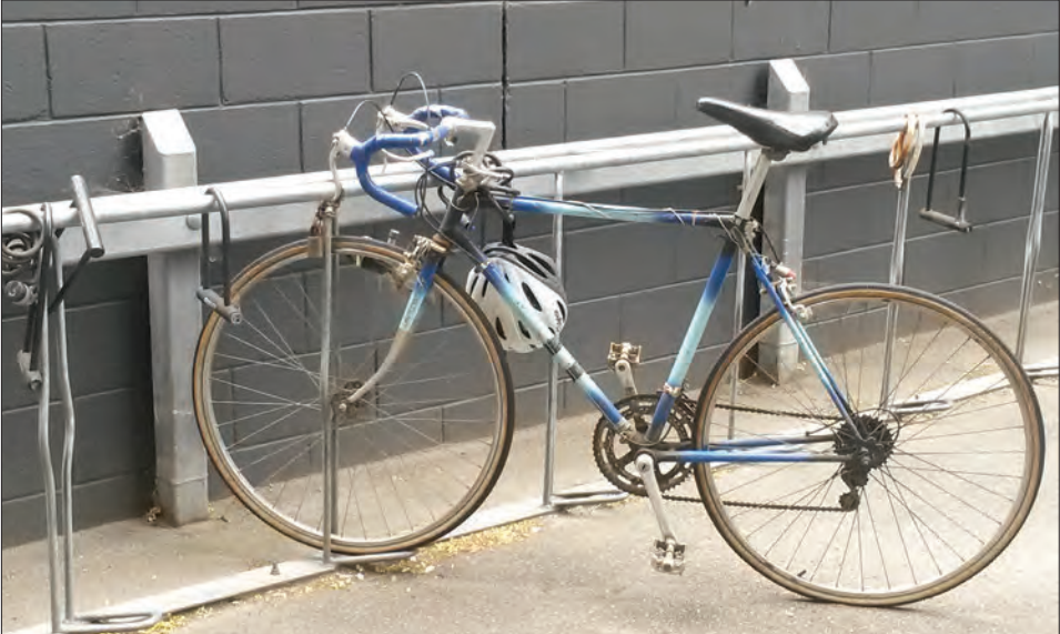
Figure 16.25: Cheap, easily installed rack that provides no frame support and can damage bicycle wheels. (Source: author's own work.)
