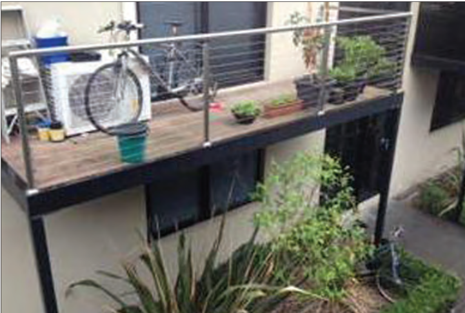
Figure 16.5: Storage requires the bicycle to be lifted up steps. (Note the bicycle behind the hedge, secured to a pole). (Source: author's own work.)
