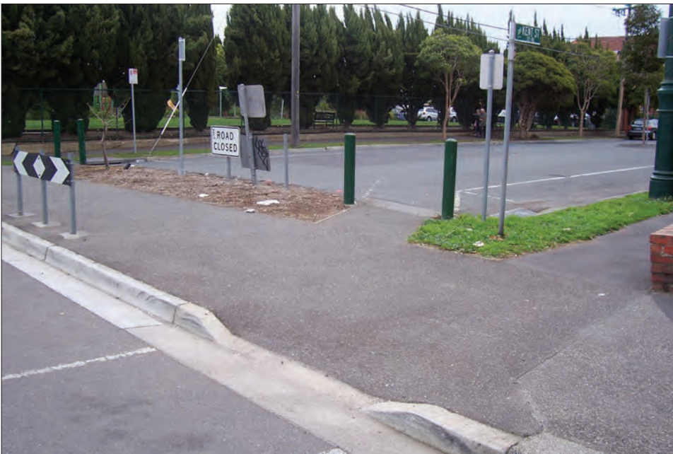
Figure 12.3: Cycle bypass of a street closure, Melbourne, Victoria. (Source: Author.)
