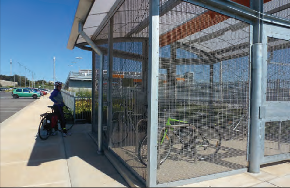
Figure 15.22: Access from the rear of the bicycle cage is unsafe. (Source: Author's own work.)
