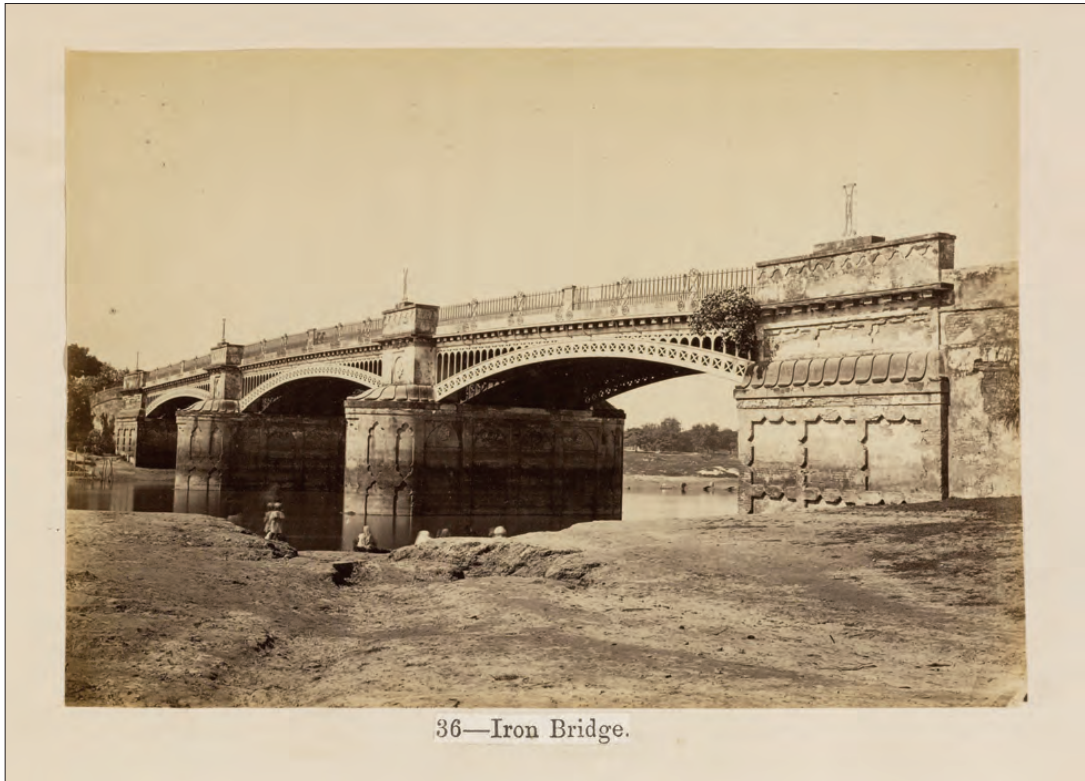
Figure 4.4 The Iron Bridge. c. 1870. Photograph by Darogha Abbas Ali. Published in The Lucknow Album. Plate 36. Reproduced from https://archive.org/details/gri_000033125008608313 . Digital image courtesy of the Getty Research Institute. The bridge was built in 1848-50 and founded by Wajīd ‘Alī Shāh.
