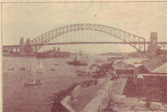
Sydney Harbour Bridge.
