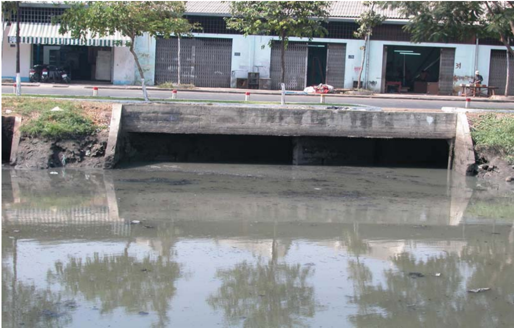
Domestic wastewater discharged directly into the Nhieu Loc-Thi Nghe Canal system, District 3, HCMC. Photo was taken by the author, February 2005.
