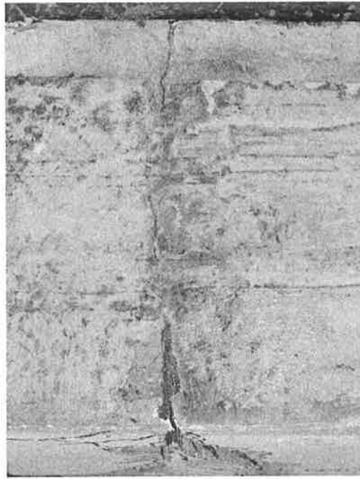
Figure 5.6.55: Splitting of concrete block for 100mm edge.
