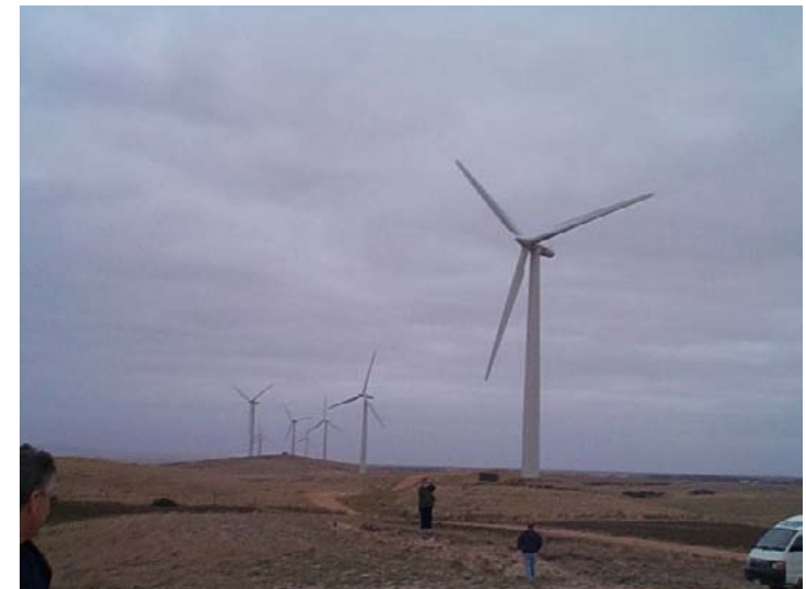
Figure 1.3 Wind farm located at Codrington, South West Victoria Source: Brett Grimm
