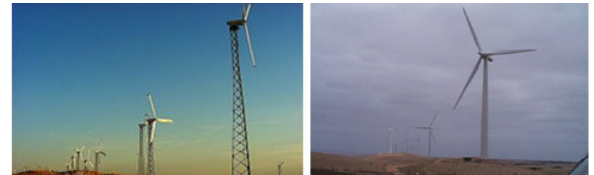
Figure 5.6 Turbines on the left are lattice towers used in New Zealand, Tararua Wind Farm (Works Consultancy Services 1995). On the right are the more common steel tubular towers; Codrington, Victoria: photo source (Brett Grimm, 2005).
