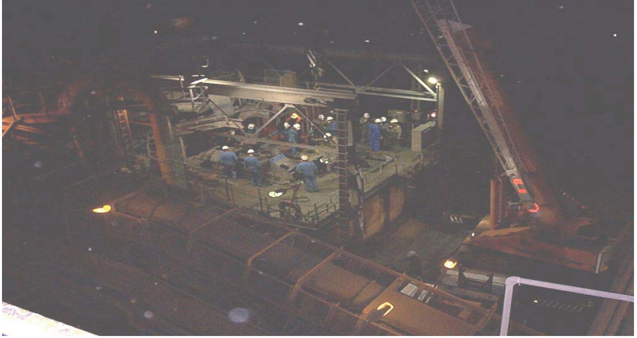
Photograph 4: Contractors on night shift conducting maintenance work
