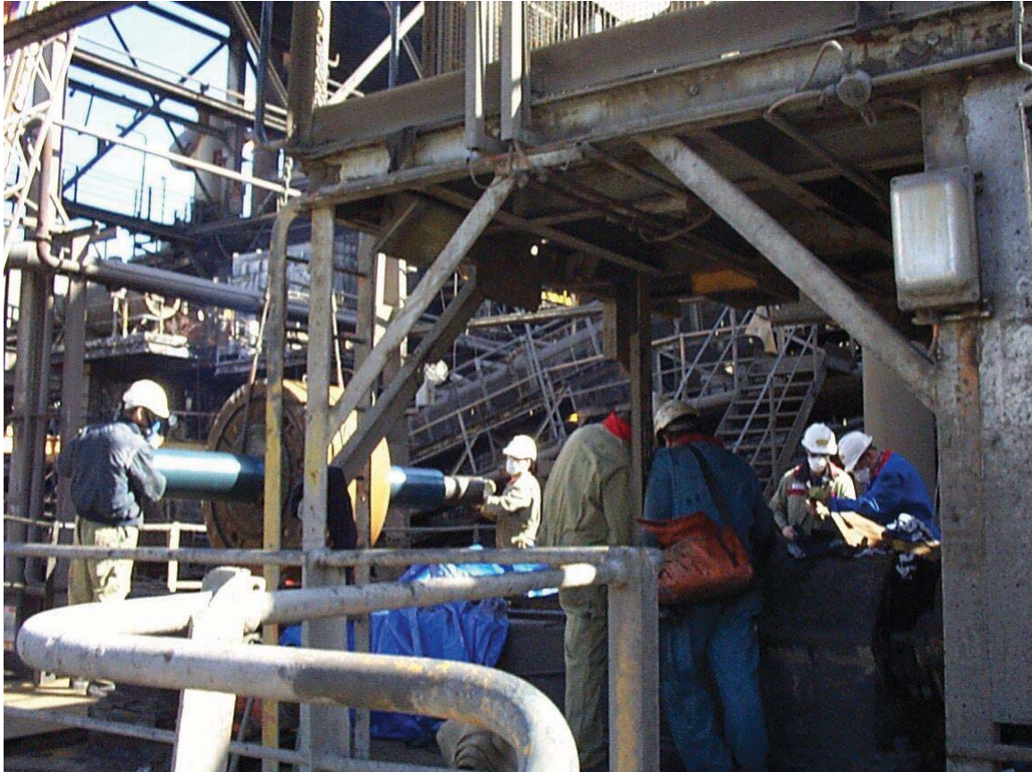
Photograph 5: Typical routine maintenance work contractors performed during day shift
