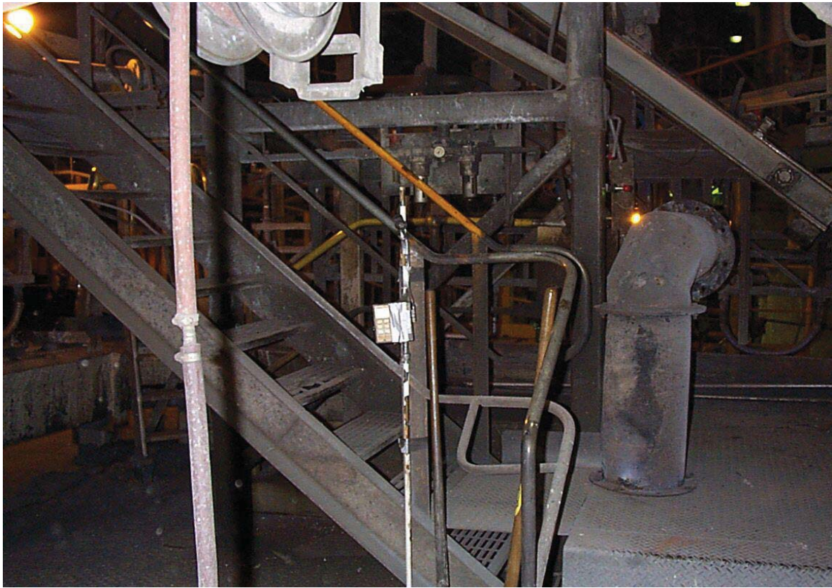
Photograph 7: Air monitoring in the area adjacent to the blast furnace
