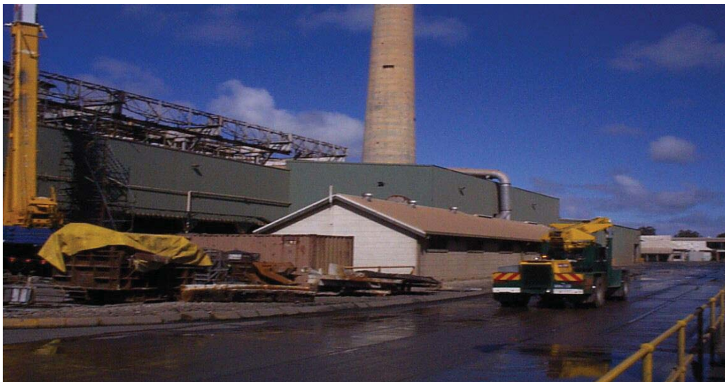
Photograph 2: Front of blast furnace illustrating the scale and size of the operation
