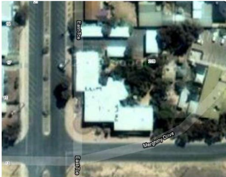
Figure 44: The Ceduna Indigenous Community Coordination Centre (the former ATSIC Building) located on East Terrace Ceduna was designed using the form of the eagle. Research in Aboriginal architecture has generally shown that there is generally little benefit in using totemic knowledge to generate a master plan. However, during consultations a number of people proudly pointed out the significance of the building to local people (Source: Google maps).
