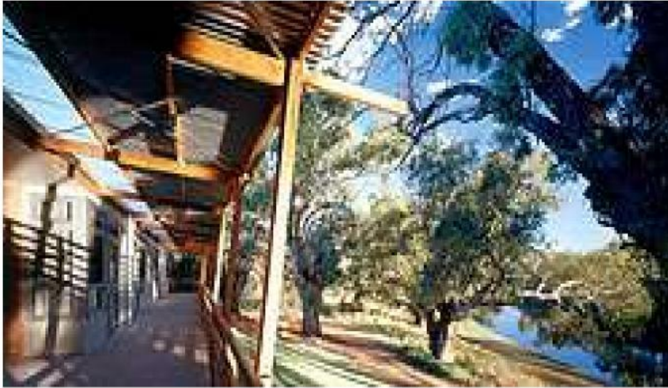
Figure 52: Wilcannia Hospital Redevelopment (Merrima Indigenous Design Unit) Architecture Australia noted “[t]he architects designed the new building as an insertion into the story of the river landscape, with tectonics developed from the river’s ‘living qualities’” (Photograph: Power House Museum).
