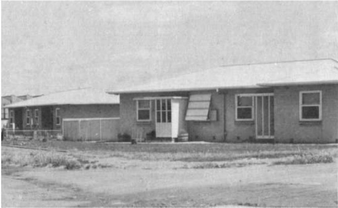
Figure 39: An example of the style of public housing by the South Australian Housing Trust commonly granted to select Aboriginal families moving from the missions and reserves to rural towns across the State. There were considerable issues for Aboriginal families living in such housing. Family sizes and domiciliary practices generally did not fit the housing type. Often this resulted in conflict with neighbours with the residents frequently experiencing racially discriminatory behaviour in the town. There was often conflict between Aboriginal and non-Aboriginal people in Ceduna. For example, Aboriginal people had separate entrances and drinking areas in all hotels in the area until relatively recently (Source: Grant and Memmott 2007).
