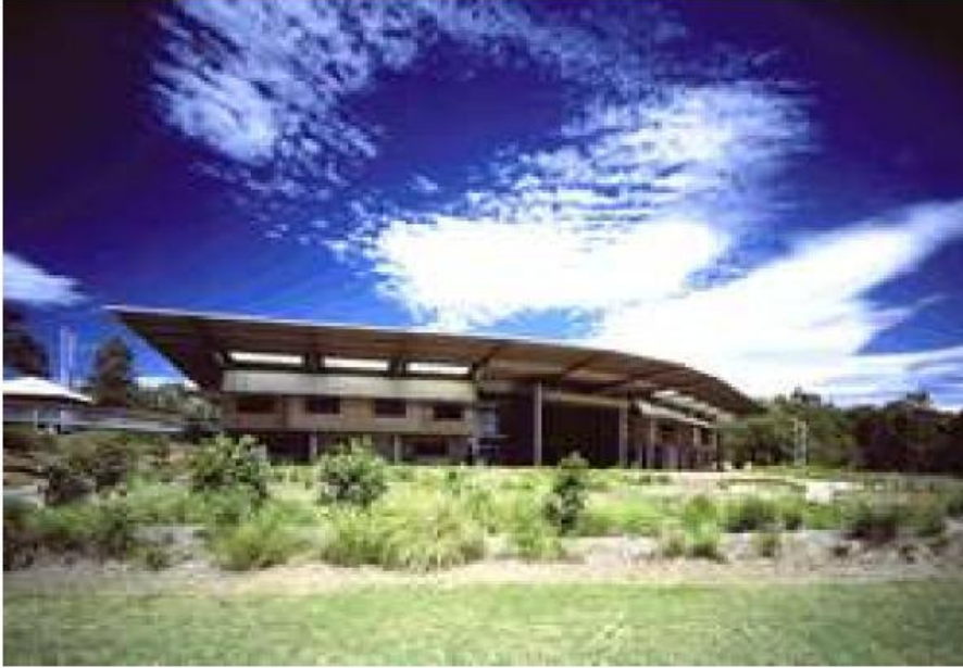
Figure 48: Gunada Centre for Aboriginal Studies, Curtin University. This Aboriginal learning centre is located adjacent to the main entrance of Curtin University in a purpose designed building. The position of the building, its architectural form and its contrast to the surrounding buildings makes a very visible statement about Curtin University's commitment to Aboriginal education and social justice outcomes (Source: http://karda.curtin.edu.au/about/place.cfm ).
