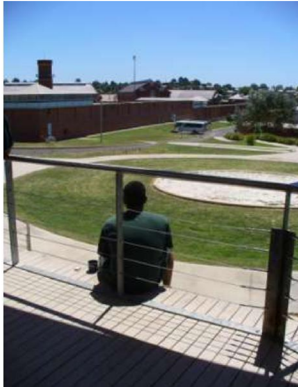
Figure 60: Decks on Girrawaa Creative Work Centre (Architects: Merrima Indigenous Design Unit) provide Aboriginal users a place to sit in the sun and observe the surroundings and provide a podium for other events (Photograph: Grant).
