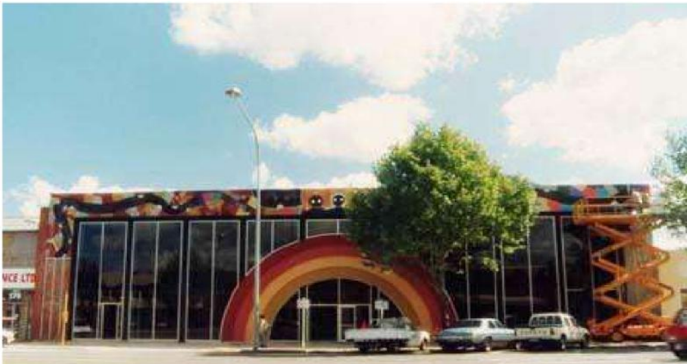
Figure 59: Nunkuwarn Yunti, Adelaide. The frontage of the building (a former retail showroom) has no signs indicating it is a community controlled health centre, but instead is decorated in specific colours and layered with symbols and icons (Photograph: Grant).
